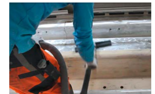
Traveller Installation SNCF Trains
